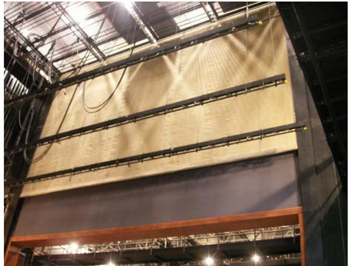
Proscenium fire curtains for theaters and auditoriums are often made with ZetexPlus® Steel™ wire reinforced fabric for extended protection in the event of a fire. The wire significantly improves the strength of the fabric which can weaken when exposed to flame. Z-Block™ Steel™ wire reinforced fabrics are often used to fabricate fire curtains for commercial buildings.
